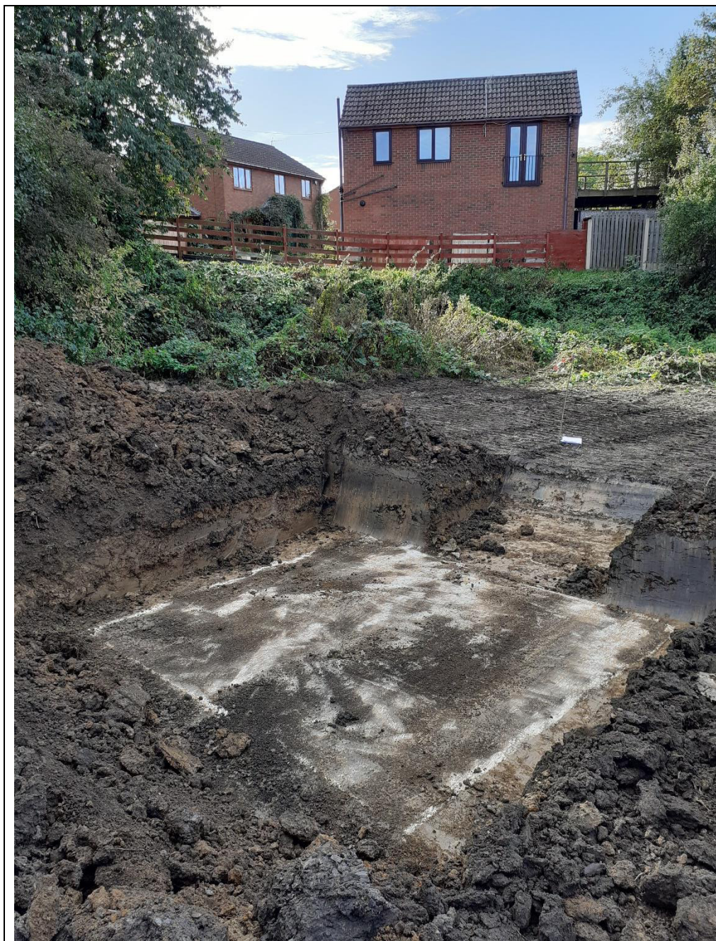
Plate 1: Concrete slab forming the cap on mineshaft 445375-014.
